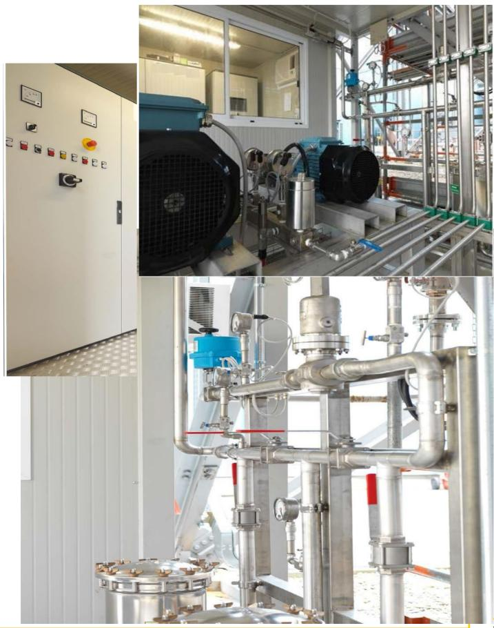
Wet Compression technology is the most cost effective and currently specified power enhancement technology for gas turbines. The concept consists in applying cooling to the air feeding of the gas turbine compressor. Demineralised water is injected into the intake airflow in the form of a fog of fine water droplets <5 micron for the nozzles installed.
