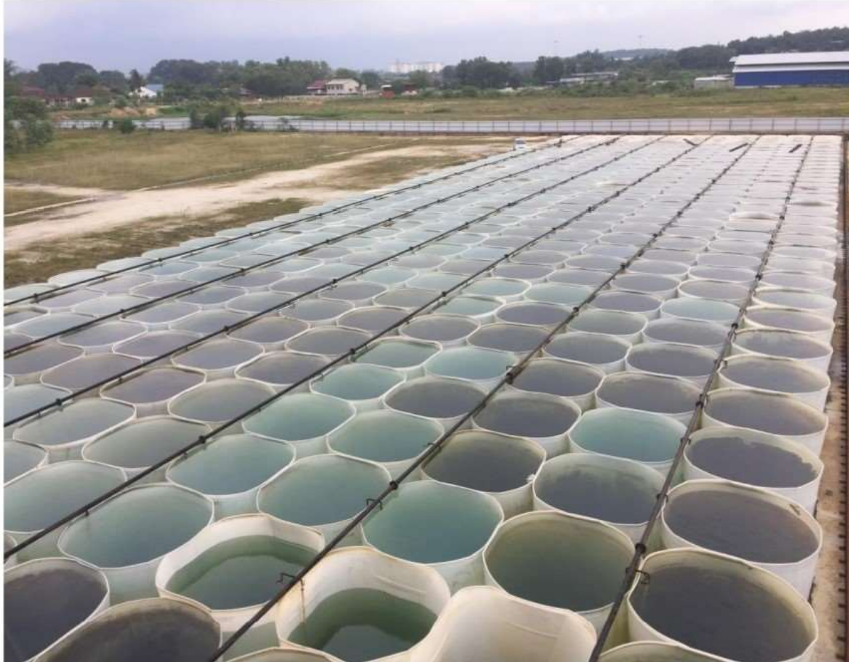
Modular Installed Tanks With Aeration Lines Installed
